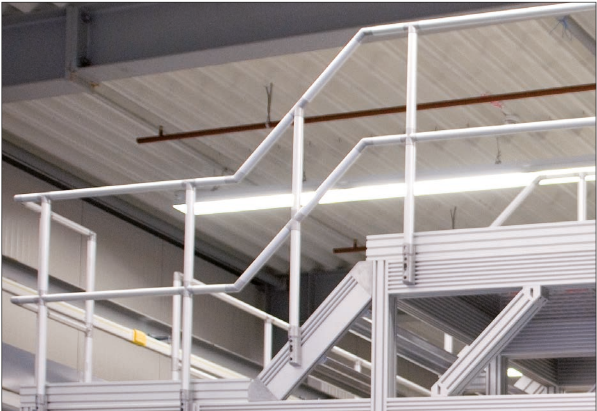
Staircase between two operating platforms.
