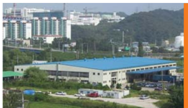
→ Head Office and Factory - 1
