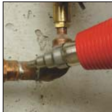
Solder Copper Pipe
