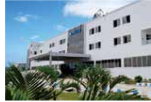
Rudrapur Plant (Green Building)
